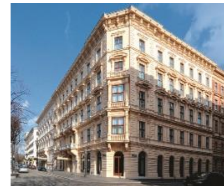
The Ritz-Carlton, Vienna, A-Wien Operador: Ritz-Carlton-Gruppe Inversor: Verry Capital, KZ-Kasachstan
